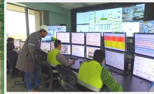
Pipeline - Control Tower
